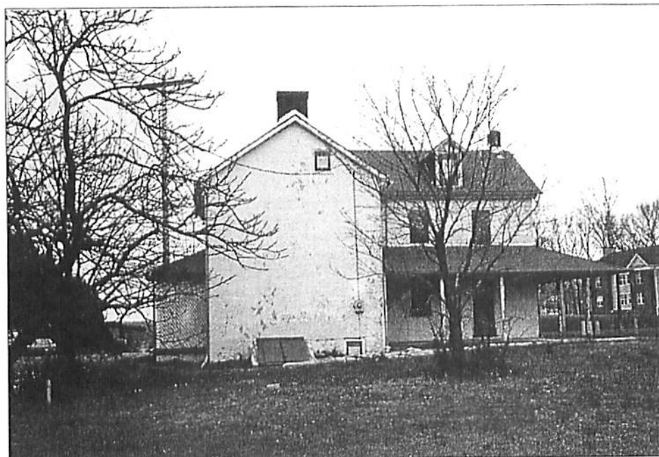
Figure 4. East elevation, the George Murphy House. View of the original stone portion of the structure and the frame addition with its wraparound wood porch.
