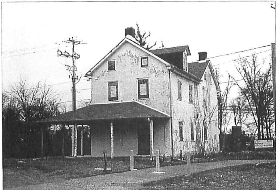
Figure 6. West elevation, the George Murphy House. The frame addition to the house is in the foreground.
