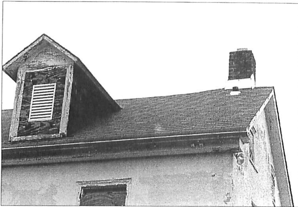
Figure 11. View of the new asphalt-shingle roof and new gutters.
