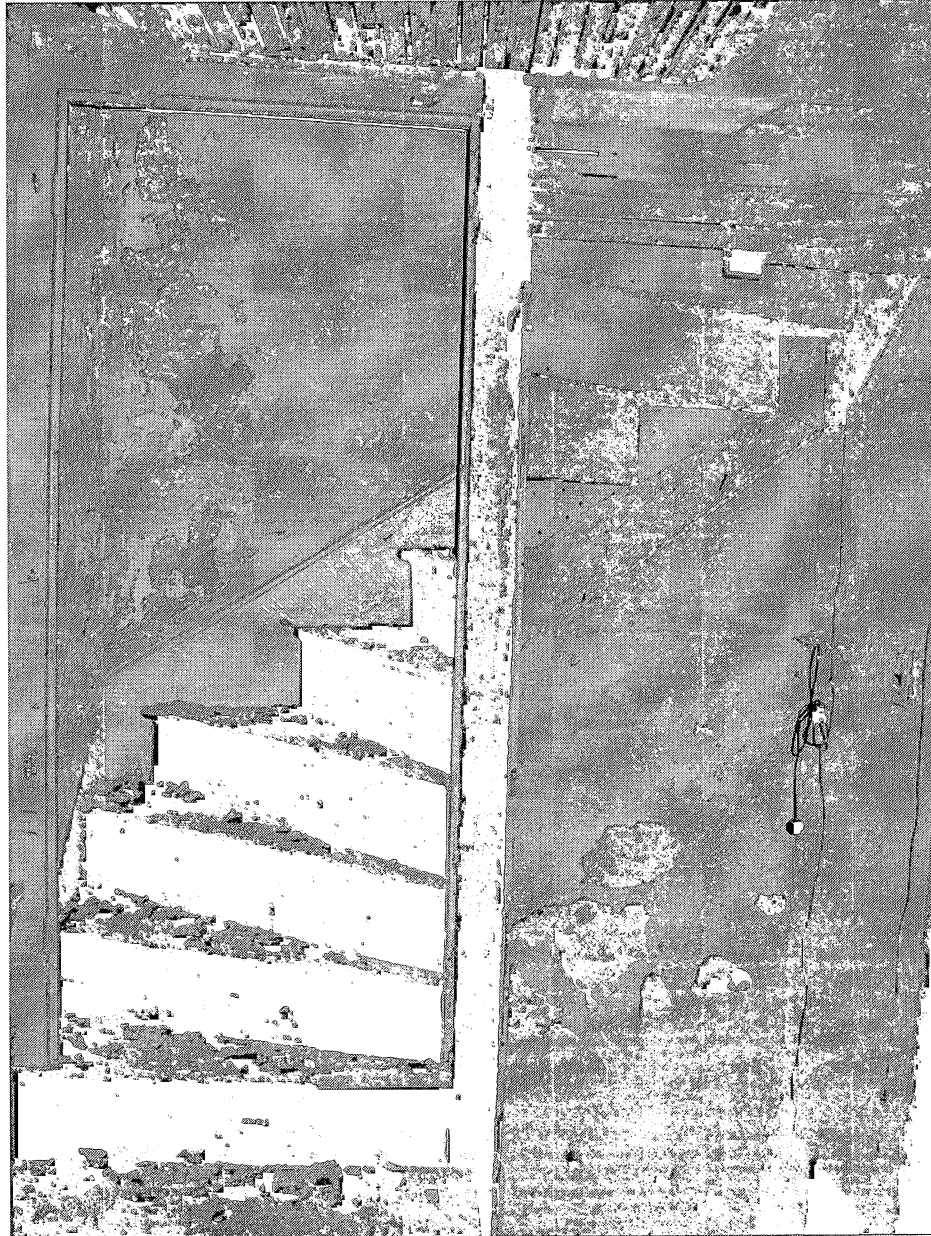
First Floor – Winder Stair
